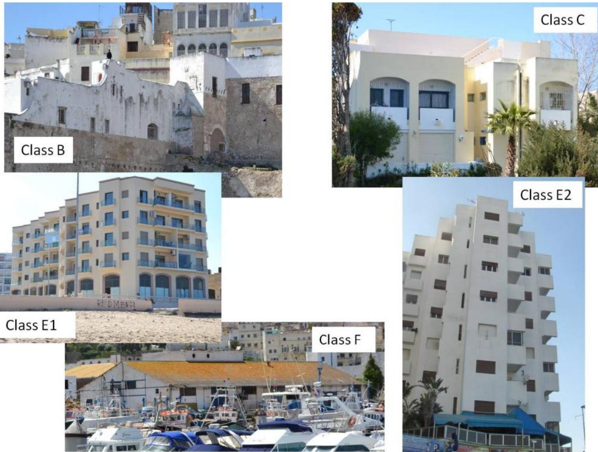
Figure 3.2.6. Examples of constructions indicating different building vulnerability classes at the city of Tangier.
