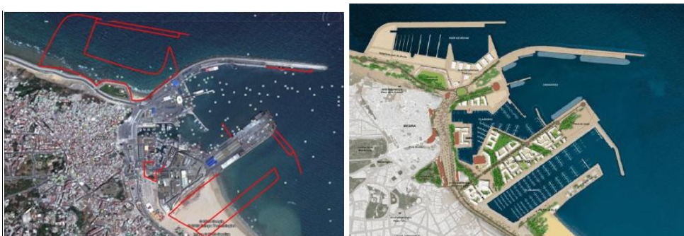
Figure 3.2.2. The Tanger harbor: Before / After
